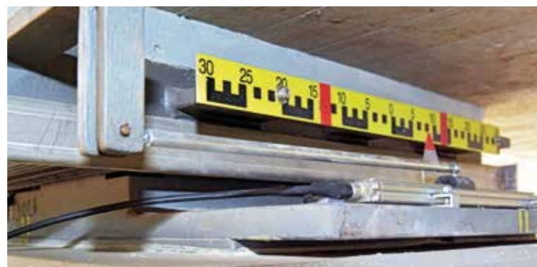
Spherical sliding bearing KGA with displacement measuring
