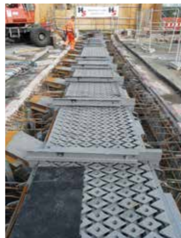
The new expansion joints are noise-reduced. When crossing the roadway expansion joints, you will not recognize any difference to the road surface.
