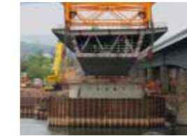
The new Schiersteiner Bridge under construction
