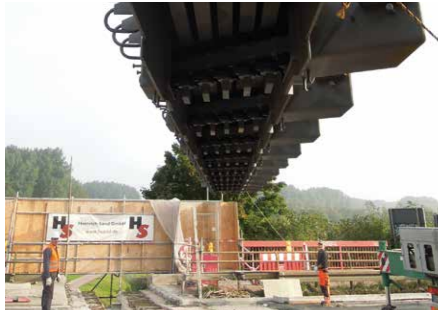
Delivery of the expansion joint
