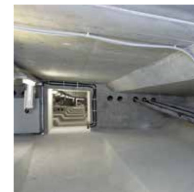
Instrumented bearing at axis 40. On the right: view into the box girder of the bridge, in the foreground sensor cables
